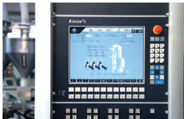
Fig. 3. Centralised touch-screen monitor of the control unit
