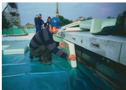
Fig. 2. CO 2 as a blowing agent – XPS insulation sheets for the construction industry (photo: BASF)
