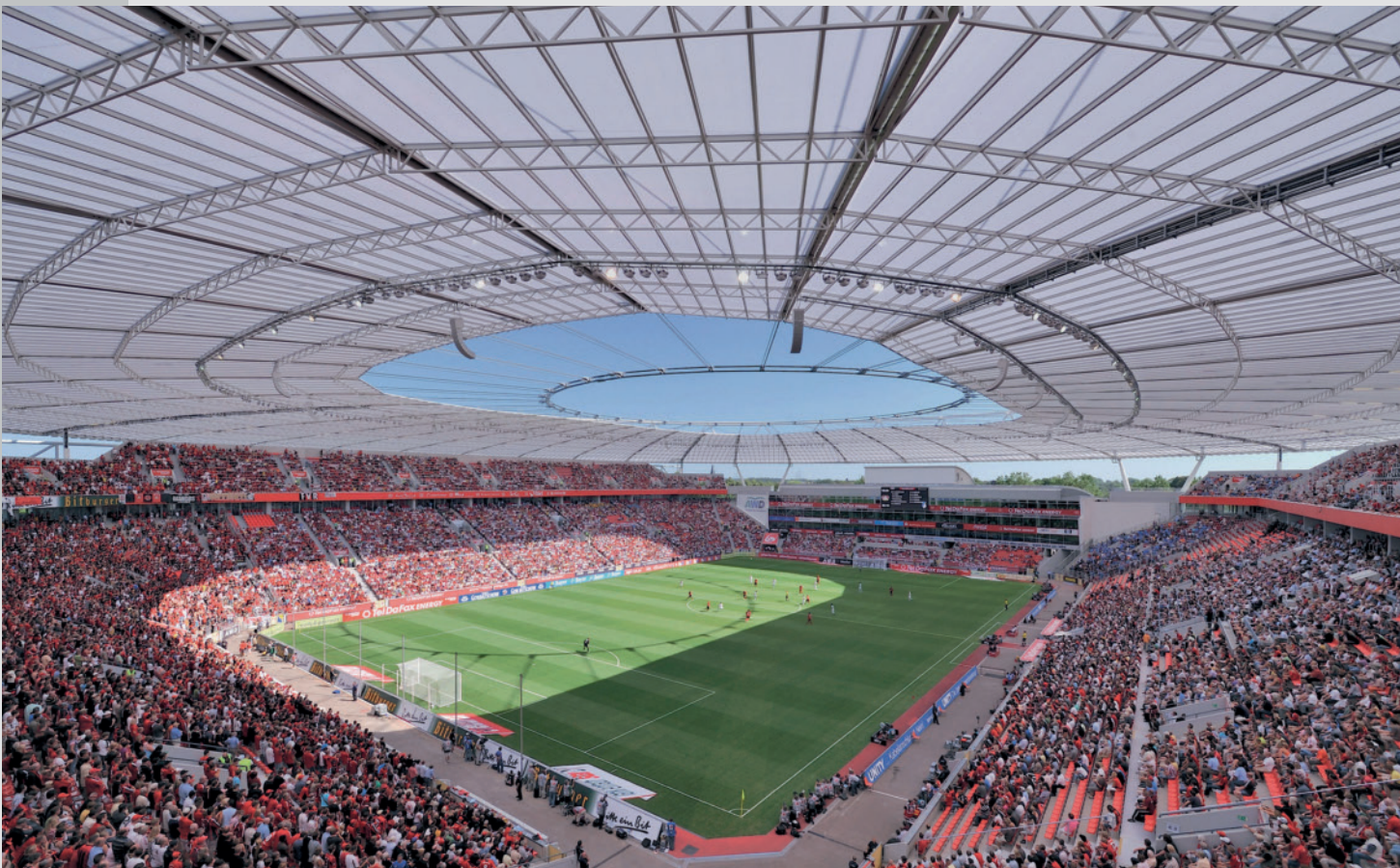
Roofing design for the BayArena football stadium: the roofing material is polycarbonate because of its transparency, stability, impact strength and weathering resistance (figures: Bayer MaterialScience)
