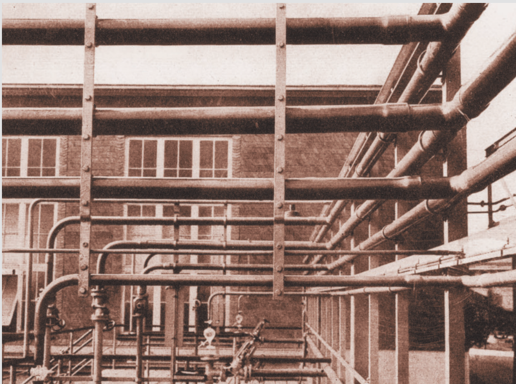
Fig. 3. "Vinidur" pipe laid outdoors (source: W. Krannich)
