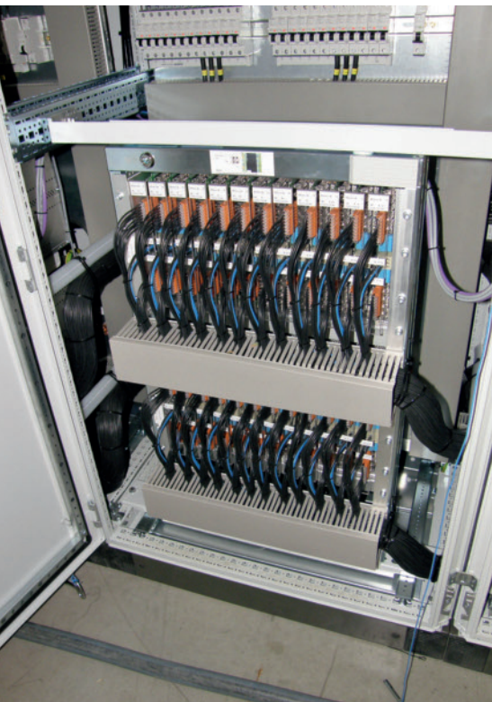
The HCS716I modular heating control unit is a key element for achieving a reproducible quality in the end products (photo: Siemens)
