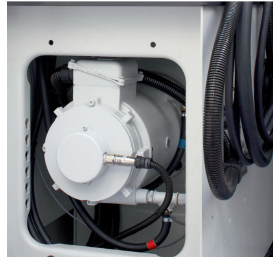
Fig. 10. Main drive – water-cooled, operated electrically and frequency-controlled – of a hydraulic injection molding machine
