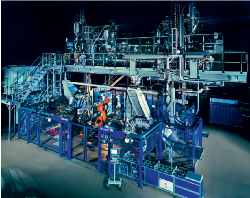
Fig. 6. Twin stations of a 6-layer, co-extrusion tank blow molding installation with robots supplying parisons for the stationary blow molds
