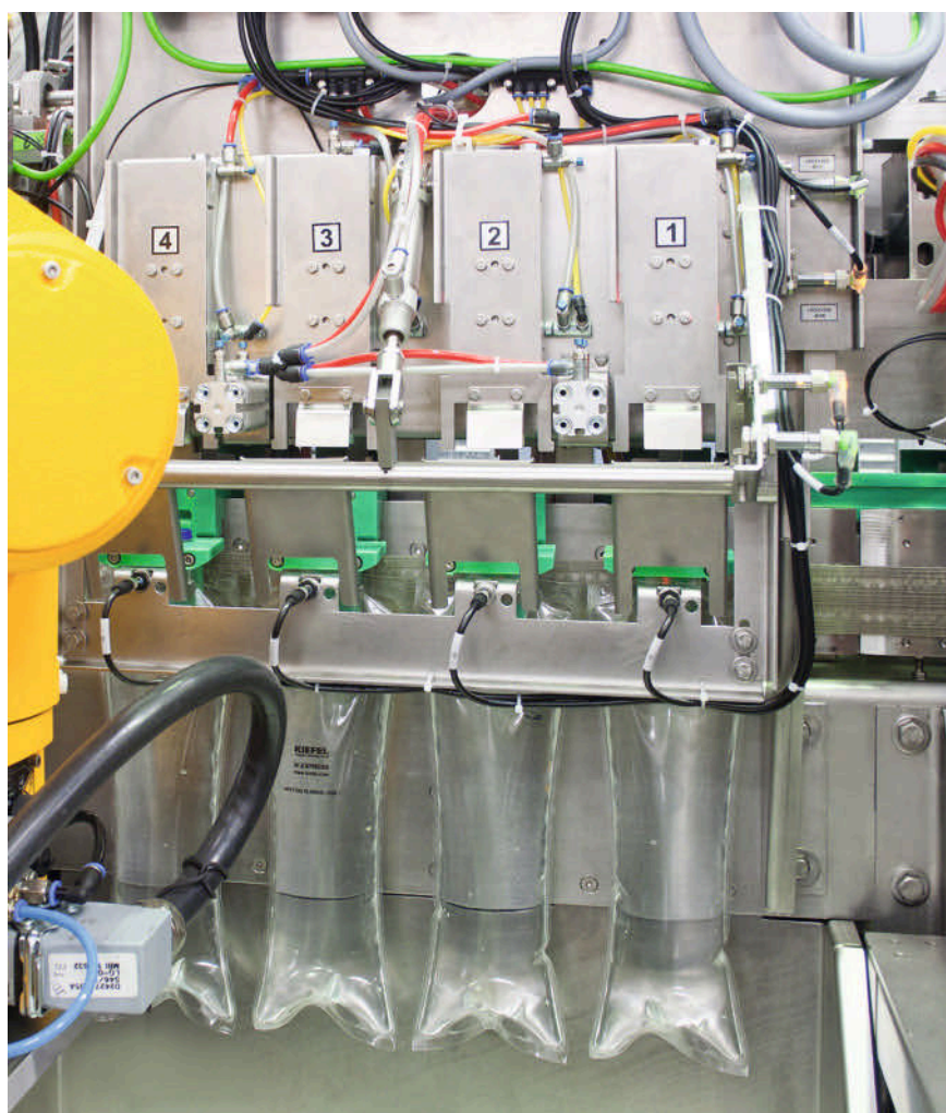
Detail of the filling station
