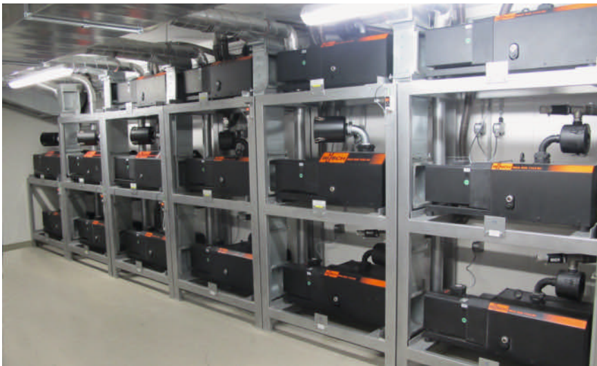
Fig. 1. Partial view of the central vacuum conveying system with Mink claw vacuum pumps at Phoenix Contact (photos: Busch)
