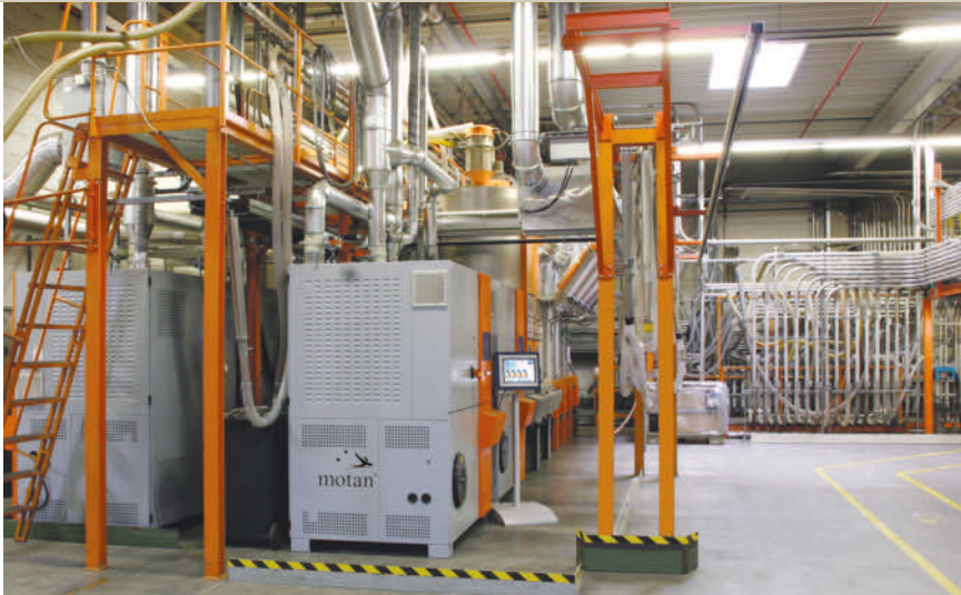
The centralized drying system supplies a variable air rate at up to 4,800 m 3 /h
