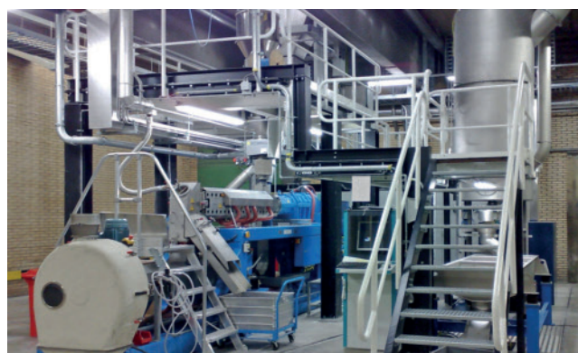
Fig. 5. Installation for the production of PVC cable compounds (photo: Buss)
