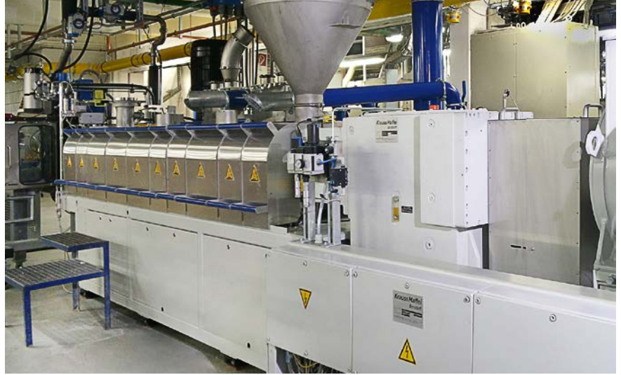
PolyComp's latest compounding line (ZE65x50D from the ZE BluePower series, manufacturer: KraussMaffei Berstorff GmbH) was installed in the first quarter of 2018 (© PolyComp)
