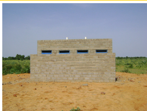
Communal latrines in Ed Daein South Darfur made with SSBs
