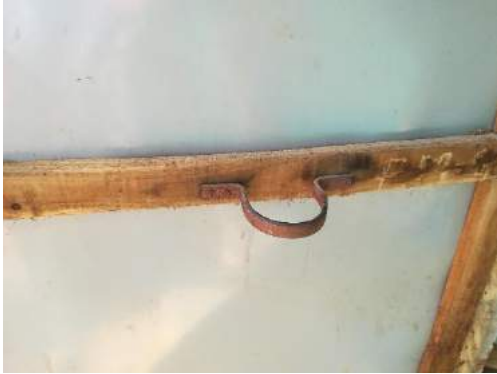
Handle use in some latrines to assist People with disabilities and elders. Photo credit: Eric Debert
