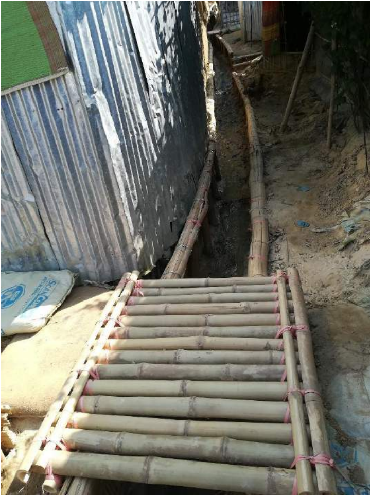
Drains constructed by the project. Photo credits@ericdebert
