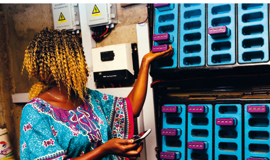
📷 Checking the MOPO batteries at a charging hub. Photo: Matt Miller/OneSixOne
