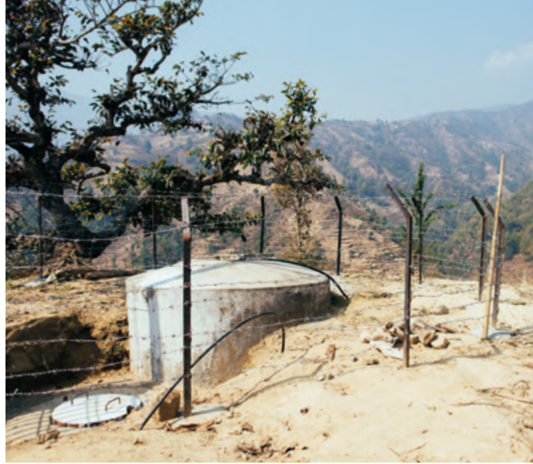
📍 This gravity-fed water tank in Nepal is protected by a fence to keep animals away from the village's water supply. A water and sanitation committee is responsible for the regular testing of the water and the maintenance of the equipment. Photo: Tom Price/Tearfund
