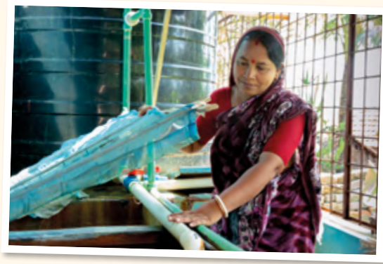
📷 Gita Roy checks equipment at the water treatment plant she helps to run.
