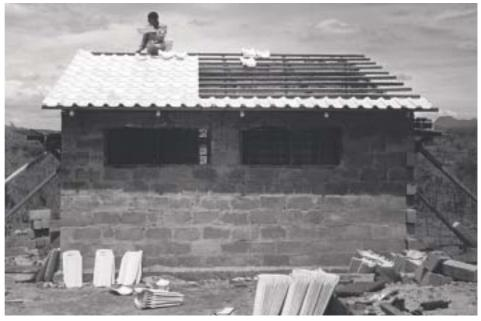
*A tiled roof needs a strong roof structure. Tiles are heavier than metal sheets. The roof will need to be well constructed with accurate measurements and level cross beams.*
