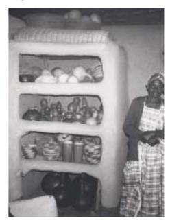
The photo shows the proud owner of an impressive-looking kitchen cupboard in Rukungiri, Uganda. Mud and cement plaster coats a wooden framework. The mat on top can be rolled down to close the cupboard.
