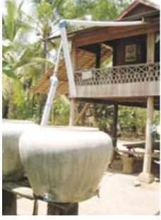
Very low cost rooftop rainwater harvesting using corrugated iron roof, hard plastic pipes and ferrocement jars for storage at a home in Cambodia.
