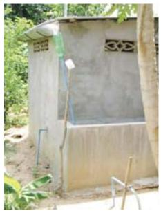
Rainwater harvesting off the roof of a latrine in Cambodia, using an old soft drink bottle, hard plastic pipe, corrugated iron and a brick storage tank. This concept is especially useful as it provides water for hand washing right at the door of the latrine.
