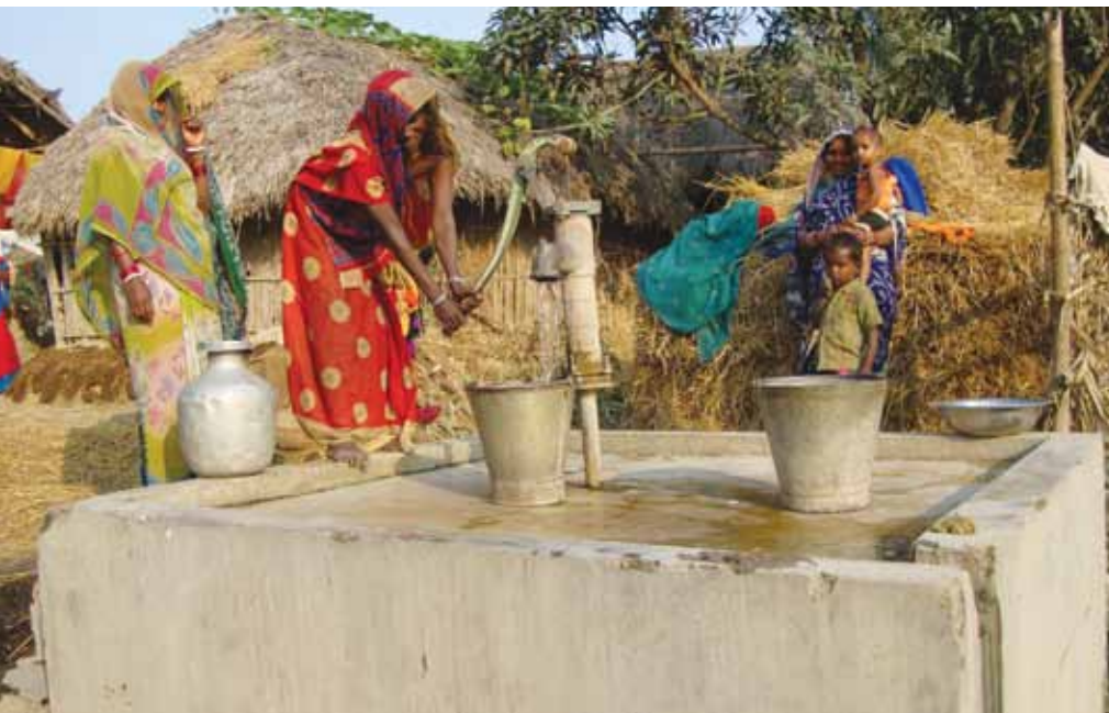
A raised tube well on a platform allows communities to access safe drinking water during flooding.
