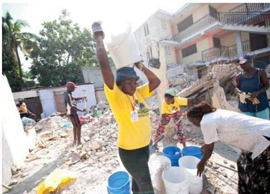
Residents of Port-au-Prince, Haiti, work together to clear the rubble following a major earthquake in 2010.
