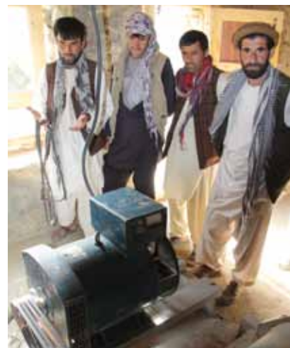
Working together on micro-hydro power projects has helped to unite communities.
