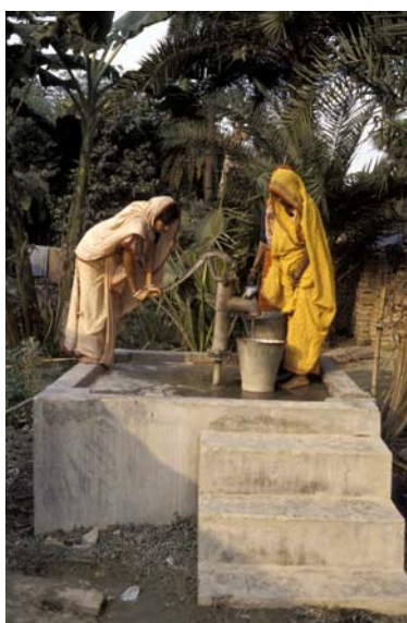
Raised platforms for hand pumps ensure that the flood waters do not contaminate or prevent access to water supply Photo: Tearfund/Caroline Irby
