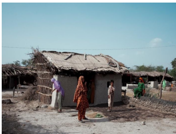
A traditional mud/straw house in Sindh villages which provide poor protection against floods
