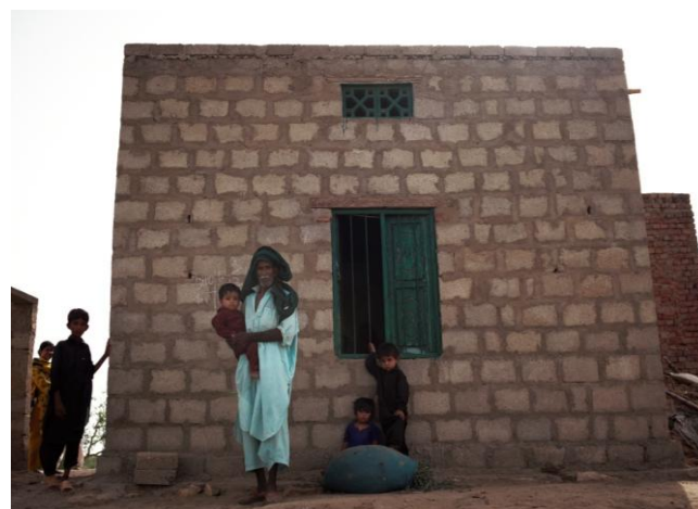
A concrete, more resilient house constructed by ActionAid in Arbab Obhayo village, Sindh
