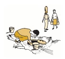
Hand-dug wells will improve water supplies in areas where natural water levels are reasonably close to the surface throughout the year. If the water level is very deep then drilling rigs will be needed. Hand-dug wells are usually between 5 and 15 metres deep and should be at least 20 metres from a latrine or
