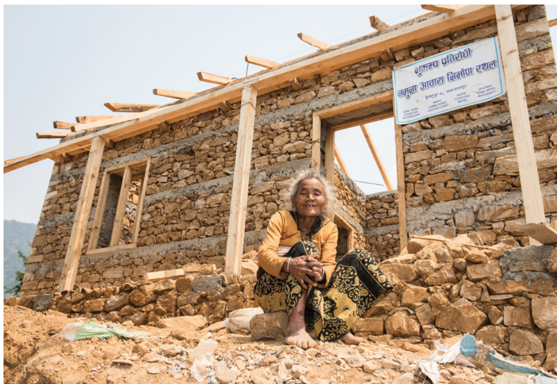
📷 A woman outside her new earthquake-resilient home, which is still under construction. Photo: Eleanor Bentall/Tearfund
