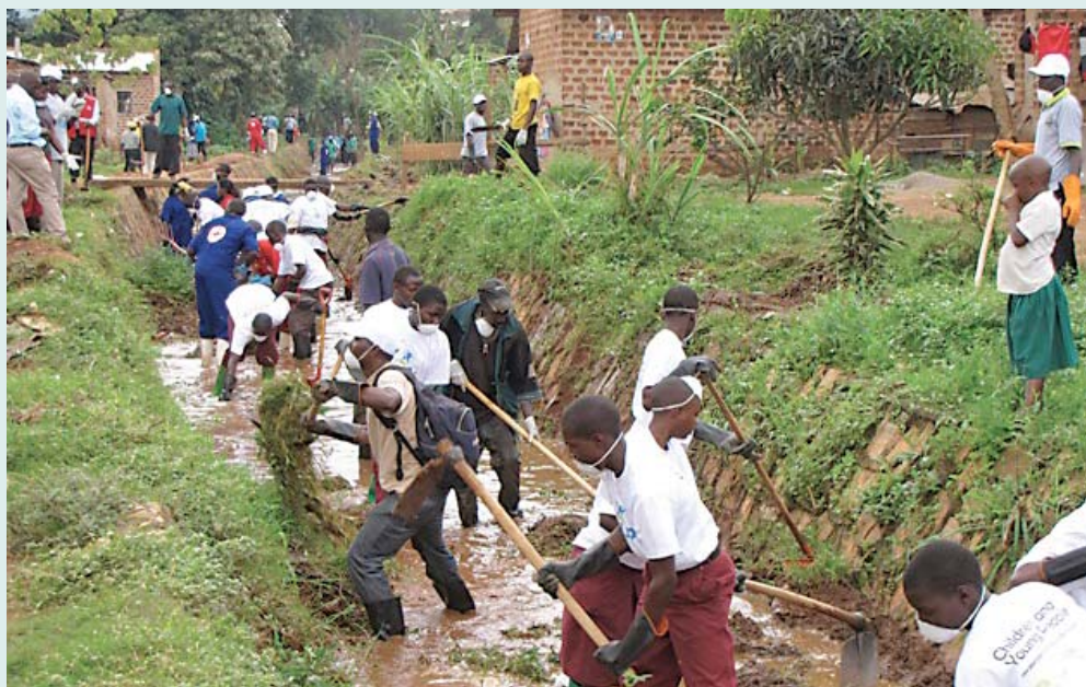
Community members de-silt a drainage channel in Kampala.
