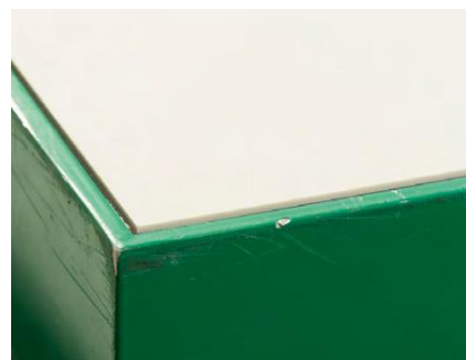
Figure 10: installed flush into the frame
