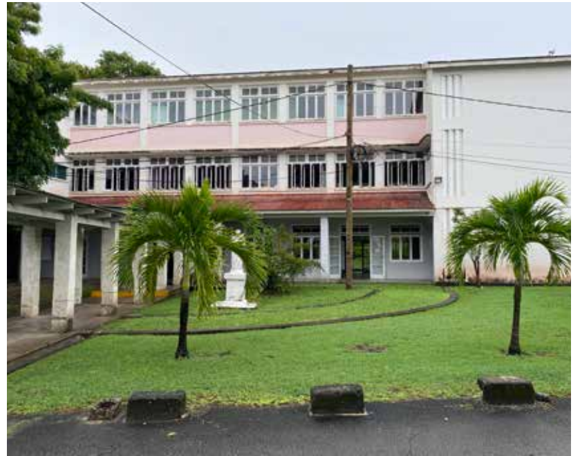
Secondary School Classroom Block
