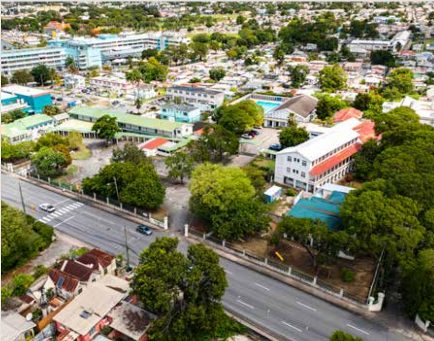
Highway 6 Entrances to The Property
