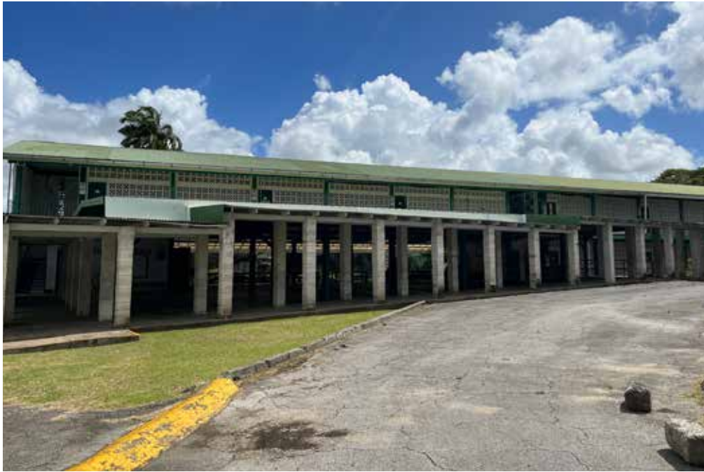
St. Angela's Covered Way and Classrooms
