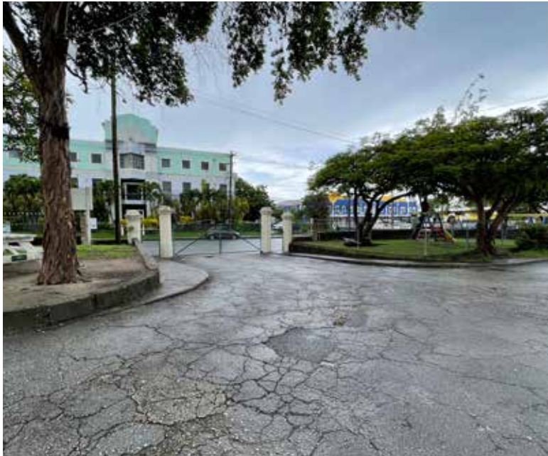
Entrance Gates Off Highway 6
