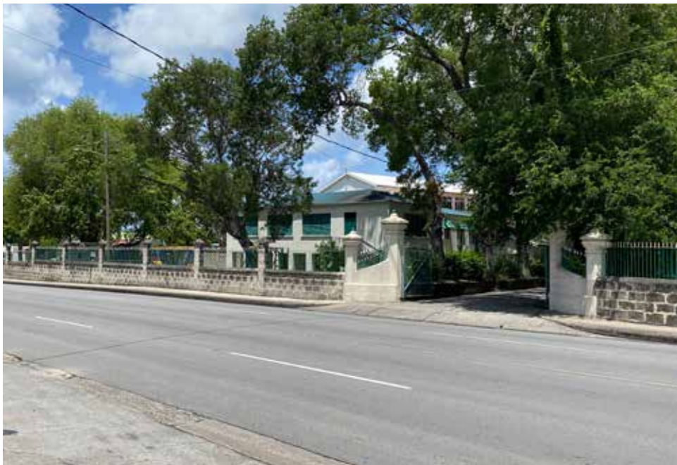
Collymore Rock, Highway 6 Eastern Property Entrance
