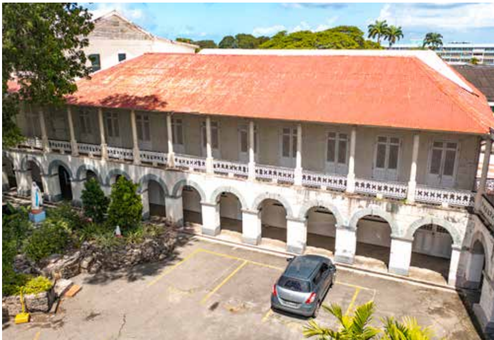
Secondary School Classrooms
