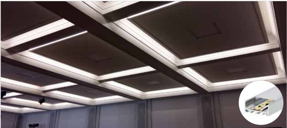
Profile: B1 Standard // LED-strips: 9,6W/m
