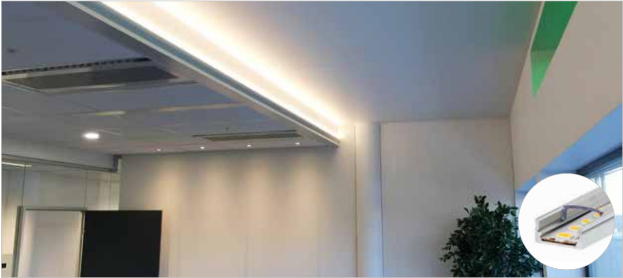
Profile: A1 Standard // LED-strips: 15W/m
