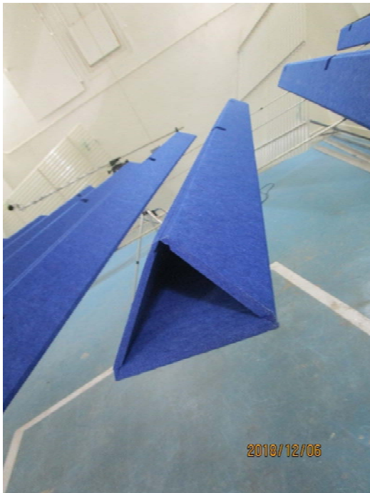
Figure 2 - Detail of individual baffle
