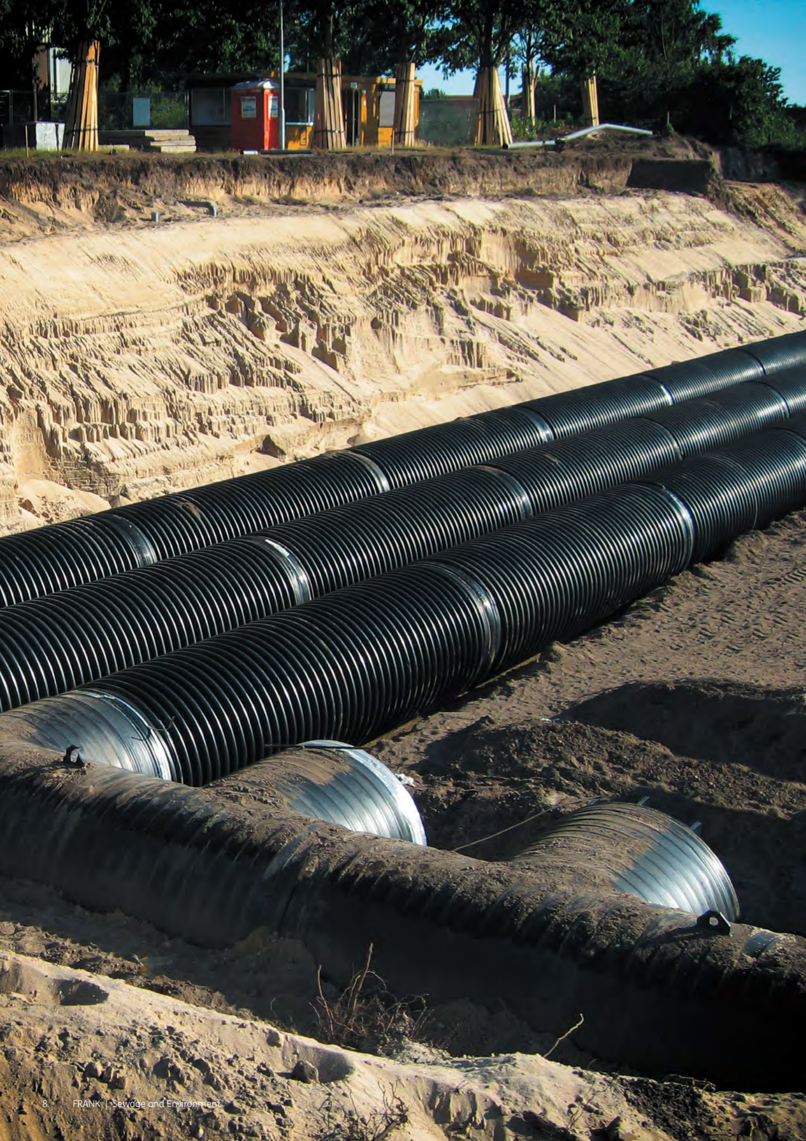
Single-pipe tank with revision chamber and two end covers
