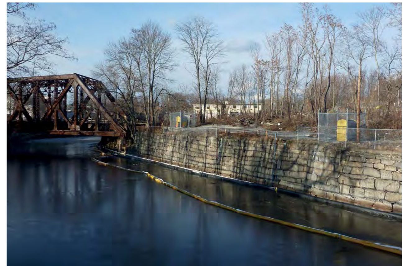
Oil absorbing curtain in water
