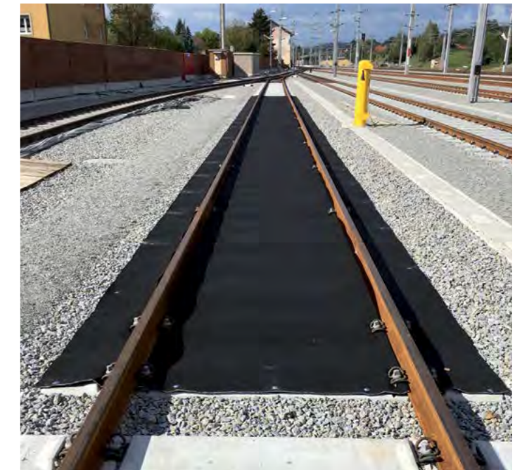
Groundwater protection for track areas
