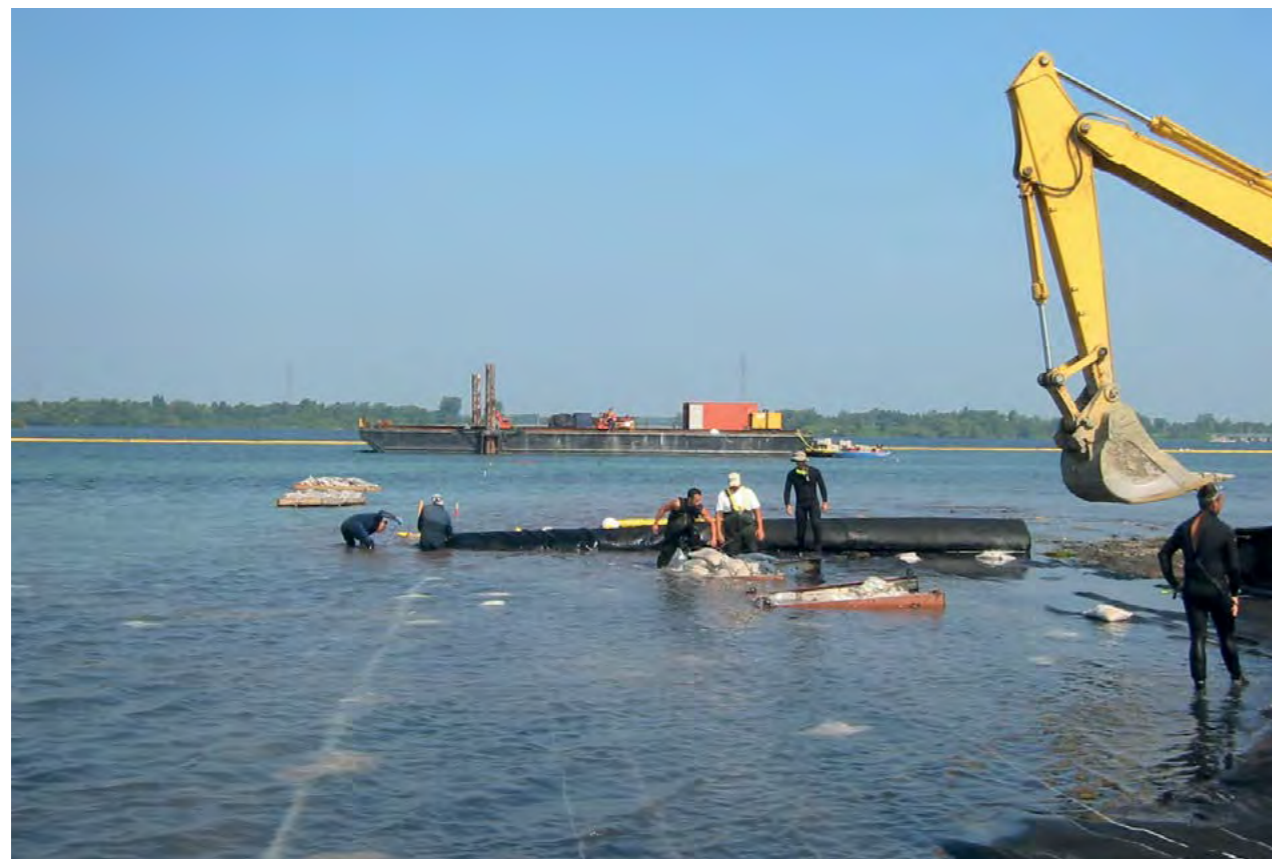
Capping of contaminated sediments
