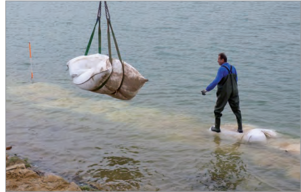
Placement of the SoilTain Bag
