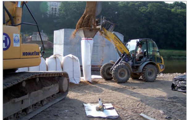
Fig. 2: Filling process of the SoilTain Bags with a funnel
