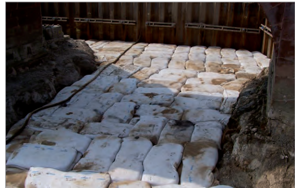
SoilTain Bags as scour protection for a bridge pier
