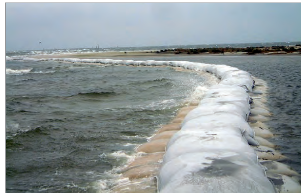
SoilTan Sand Bags for coastal protection works
