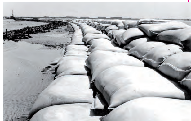
Construction of the dike core at the Rüstersieler Watt 1963
