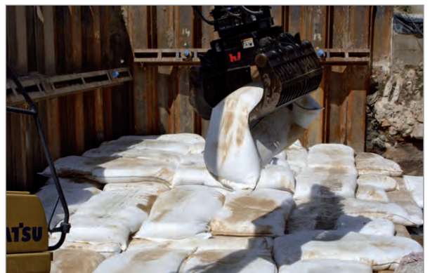
Fig. 6: Placement of the SoilTain Bags
