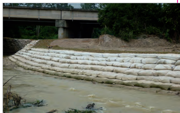
Sungai Melaka project, Malaysia in 2011
