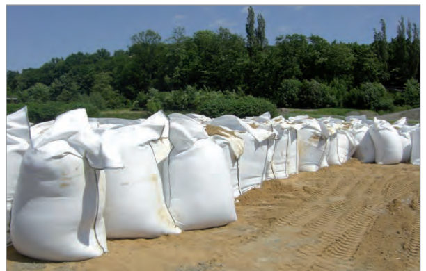
Fig. 4: Prepared SoilTain Bags, waiting for installation
