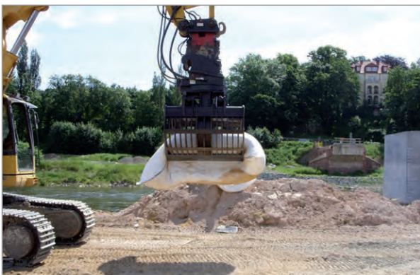
Fig. 5: Transportation by an excavator with a grab
