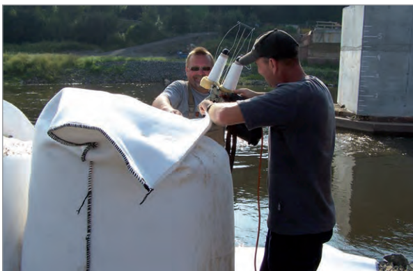
Fig. 3: Closing of the SoilTain Bags with a hand-held sewing machine
