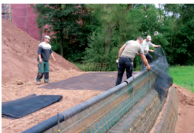
Expert installation of Fortrac® geogrids ▼
