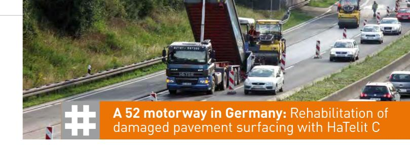
The repair works commissioned by Landesbetrieb Straßenbau NRW – the state enterprise responsible for highway maintenance in the German State of North Rhine-Westphalia – to the damaged pavement surfacing on the section of Germany's A 52 motorway between the Neersen and Mönchengladbach interchanges were carried out in July 2009 using HaTelit C. The first step was to mill off the existing surface course and binder course.
