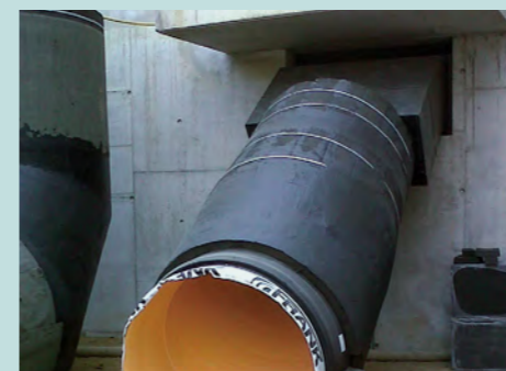
Insulated ventilation pipe with transition to rectangular building connection
