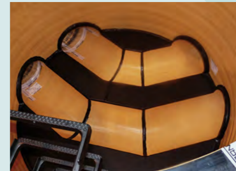
Inspection shaft with parallel angled channel
