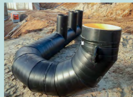
Precast segmental bend and distribution channel for ventilation
