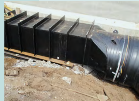
Transition of circular PKS ® pipe to rectangular duct including reinforcement
