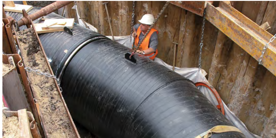
PKS® pipes compensate external forces by means of a defined deformation
