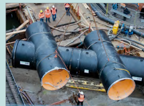
Prefabricated junction structure
