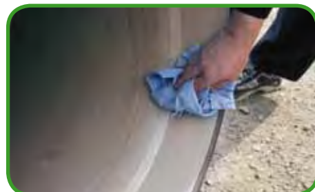
Fig. 130 - Cleaning the socket
