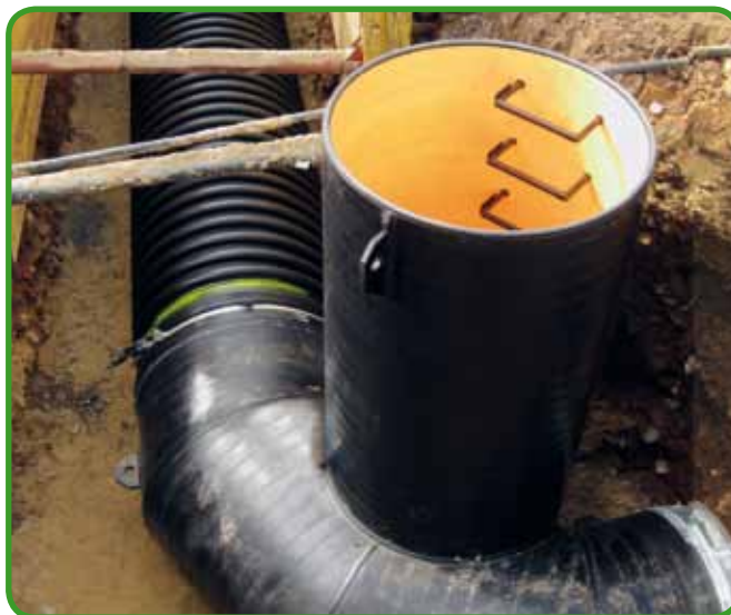
Fig. 141 - PKS® tangential manhole
