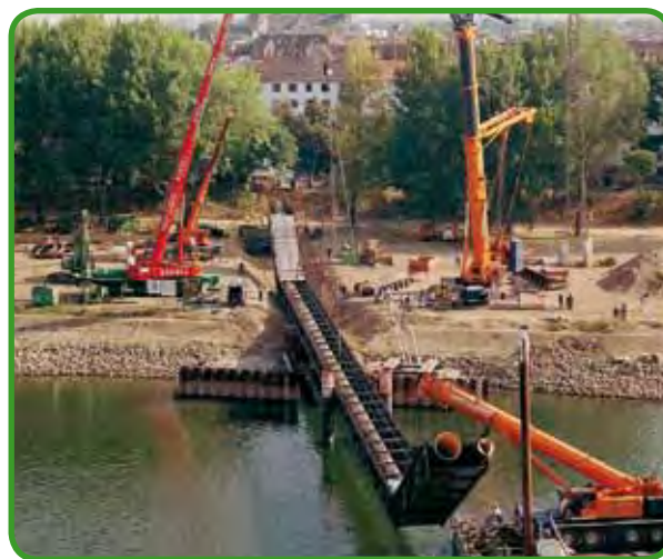
Fig. 157 - Neckar sewage pipeline prior to installation in river bed
