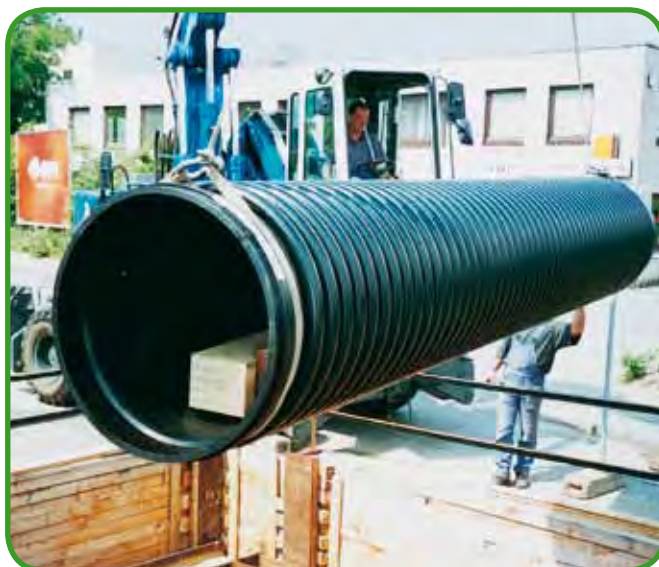
Fig. 54 - PKS® pipe with electrically conductive inside layer
