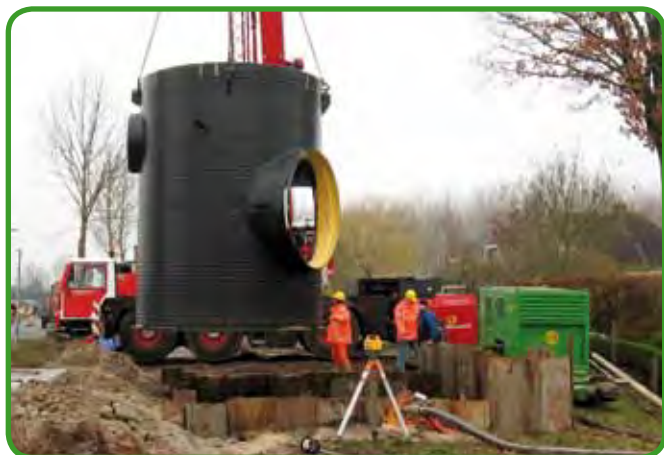
Fig. 170 - Installation of DN 3000 overflow/pump shaft
