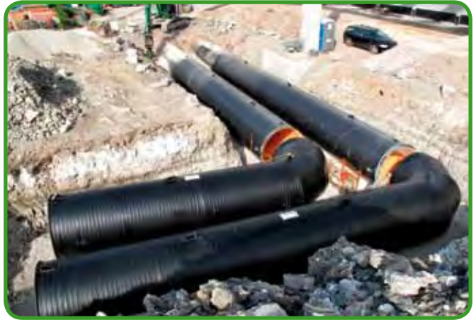
Fig. 151 - PKS® Secutec DN 2000 (DN 2000 storm water system with leakage monitoring, DIBt-approved)
