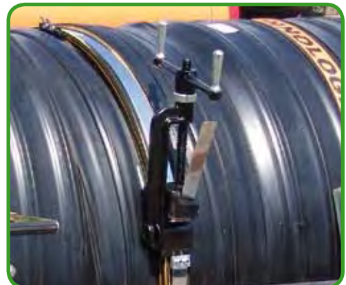
Fig. 102 - Tightening of tension bands
