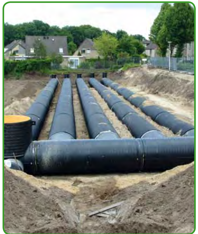
Fig. 143 - PKS® DN 1500 storm water system
