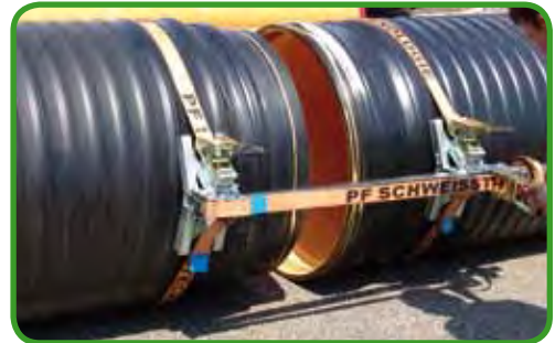
Fig. 101 - Pulling the pipes together
