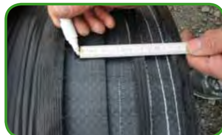
Fig. 129 - Marking the insertion depth
