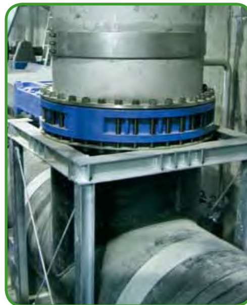
Fig. 135 - Flange connection to PKS® pipe
