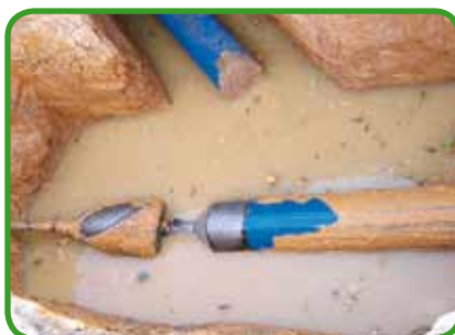
Fig. 87 - Horizontal hydraulic drilling
