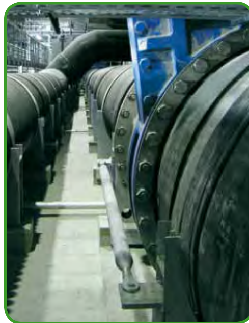
Fig. 134 - Flange connections in sewage treatment plant
