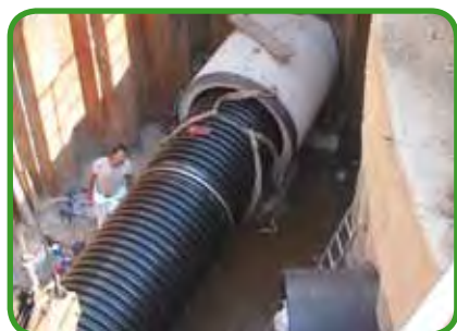
Fig. 86 - Short pipe relining
