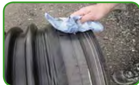
Fig. 128 - Cleaning the spigot end
