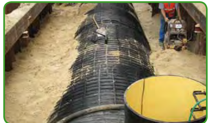
Fig. 77 - Compacting of side bedding
