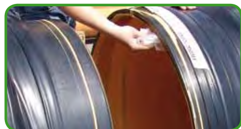
Fig. 99 - Cleaning the electrofusion socket and the spigot end
