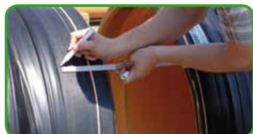
Fig. 100 - Marking the insertion depth
