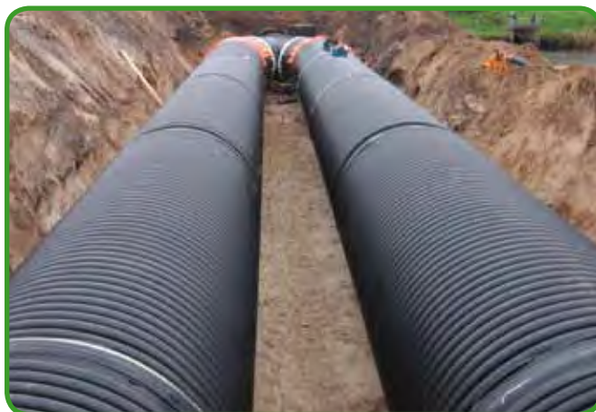
Fig. 168 - Two DN 1800 pipe strings of 78 m in length, installed between the road and a pond
