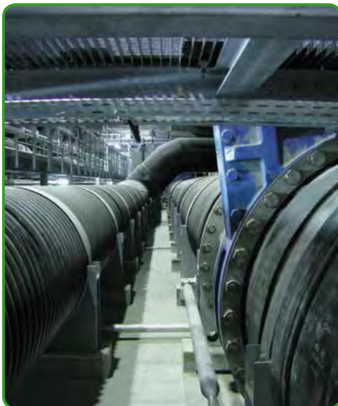
Fig. 165 - PKS® pipe flange connections
