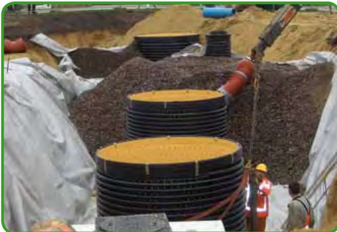
Fig. 148 - PKS® infiltration manholes
