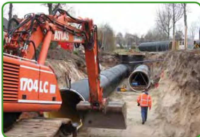
Fig. 167 - Installation of PKS® pipes
