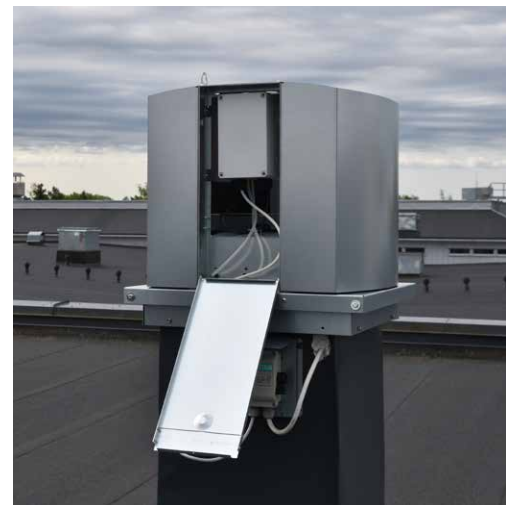
The control equipment is fully integrated inside the roof fan behind a safety door.
