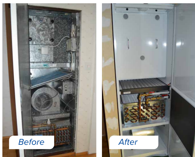
The galvanized surfaces of the interior of the old air heating unit (left) had become coarse and tarnished over the years. The new air heating unit (right) is completely painted, helping to keep the unit clean. Filters are also better today. The ventilation part features the latest technology in the industry.
