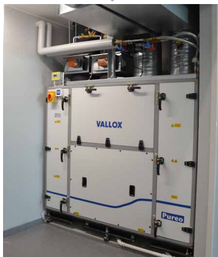
A Vallox Pureo unit with built-in automation was selected for the site as there was no existing house automation system.
