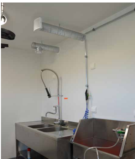
Extractions at the site ensure that potential harmful substances and steam from washing gear are efficiently extracted from the premises.
