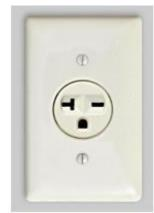
This is the 6-20R <u>Nema</u> Outlet that is needed for the plug that comes on the unit.
