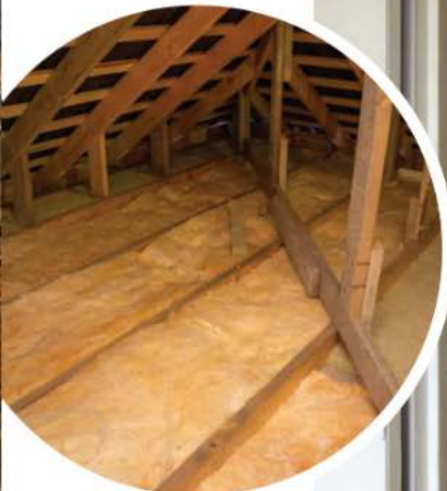
Mulberry Estates insulated its attic (above) and replaced boilers and water heaters (right).
