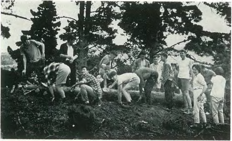
Timber for the Hut.
