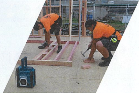
Floor Laid and Frames being Stood
