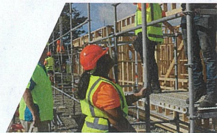
Scaffolding and Safety Net Installation by Students
