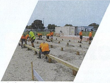
Sub-Floor and Frame Construction
