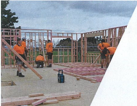
Frames being Stood and Squared
