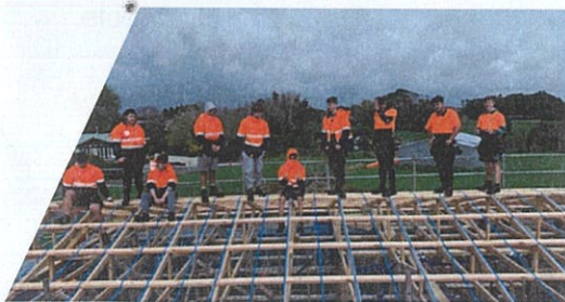
Trusses and Roofing
