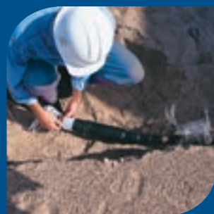
Medium Voltage (up to 33 kV) QS2000E Joint Kits
