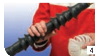
4 Once the inner core has been fully removed, the termination installation is complete!
