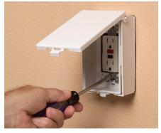
2 Install wiring device per manufacturer's instructions, and Local and National Electrial Codes using the pre-drilled holes in the base.
