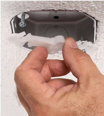
**1** Attach the bracket to the box with #8 or #10 screws. Back the screws in the box out just enough to slip the bracket on.
