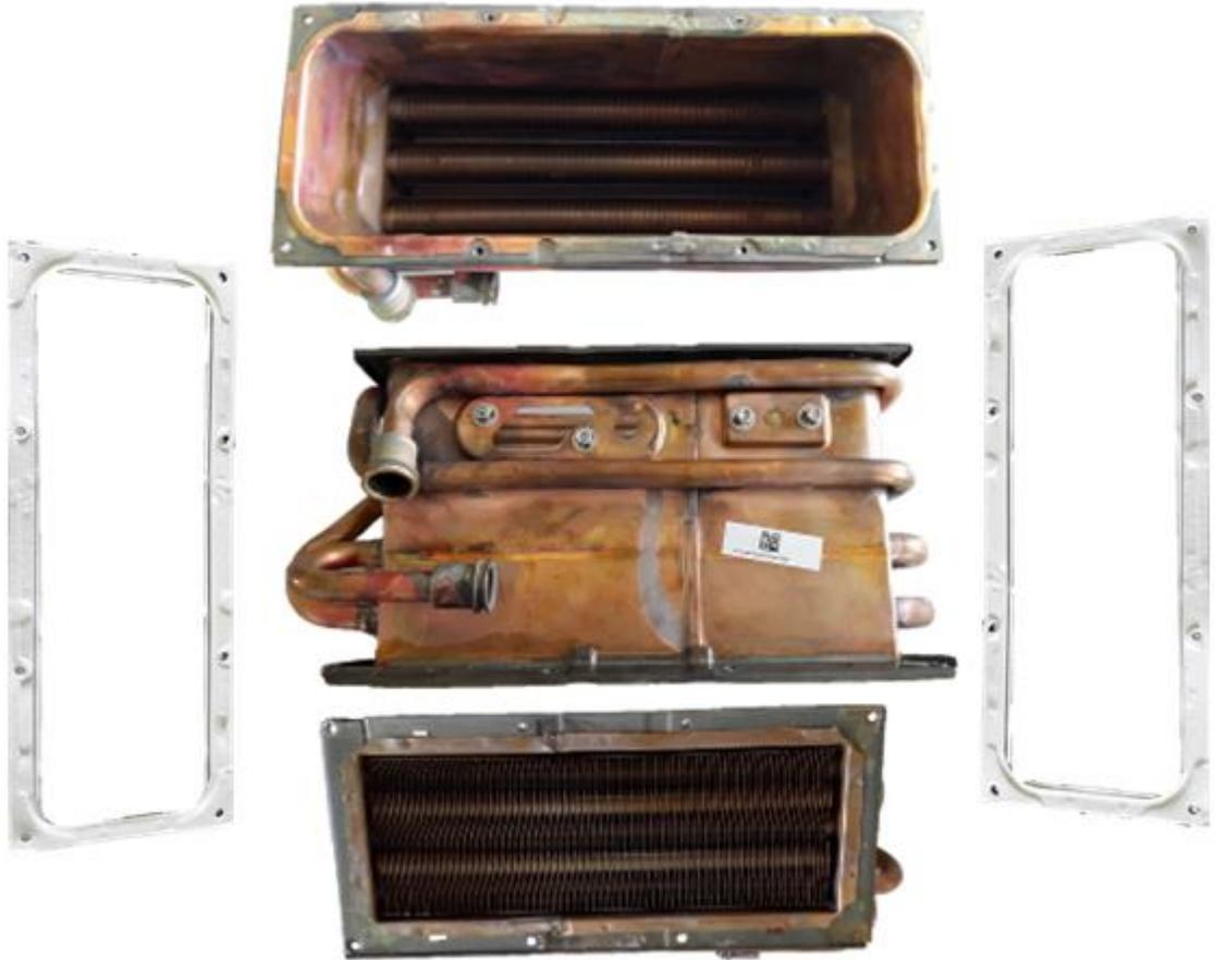
**Figure 22 – Heat exchanger**
