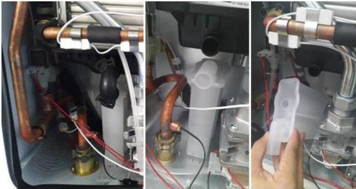
Figure 13 – Disassembling the Condensate Siphon from the Unit
