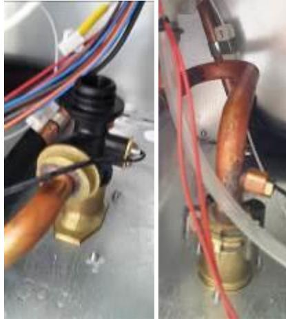
Figure 29 – Outlet Water Temperature Sensor (left) and Inlet Water Temperature Sensor (right)
