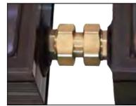
The 1¼" male union threads on the StarMax 4 collector have a flat sealing surface. The NAS10478 double union allows the collectors to be joined close together, but still allows for a collector to be removed from an array without moving the adjoining collectors. The double union has pre-installed high temperature silicone O-rings which seal against the coupling flat surface and will not fallout during coupling. This provides fast torch free connections.
