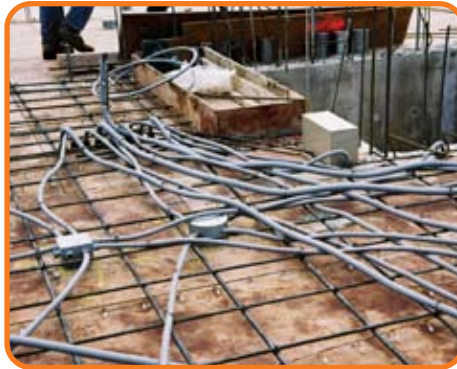
Diagram 3. ENT is tied to the rebar in intervals.
