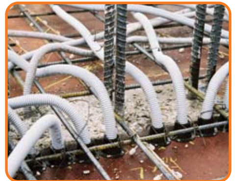
Diagram 4. ENT is bendable and flexible.
