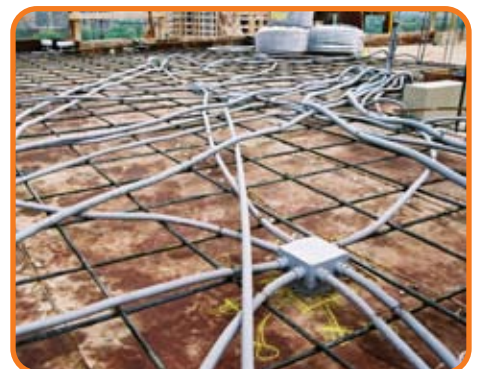
Diagram 5. Ident-A-Box™ with Hub Extensions.
