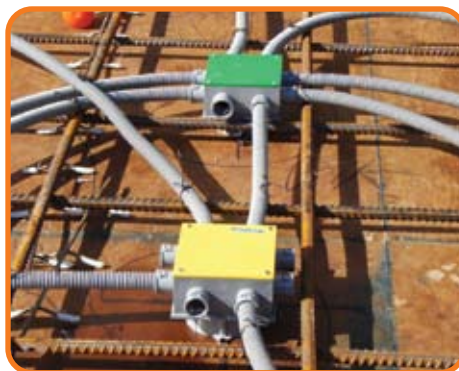
Diagram 5. Colour coded lids for easy electrical identification.
