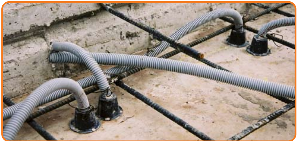
Diagram 1. ENT encased in a concrete application.
