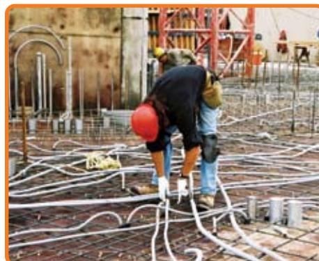
Diagram 2. ENT and fittings in a High-Rise application.
