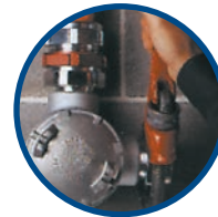
5. Install hub on enclosure
