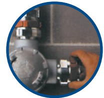
6. Insert cable and tighten red union
